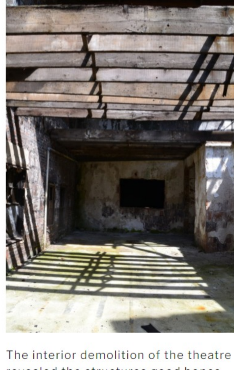
The interior demolition of the theatre revealed the structure's good bones.
