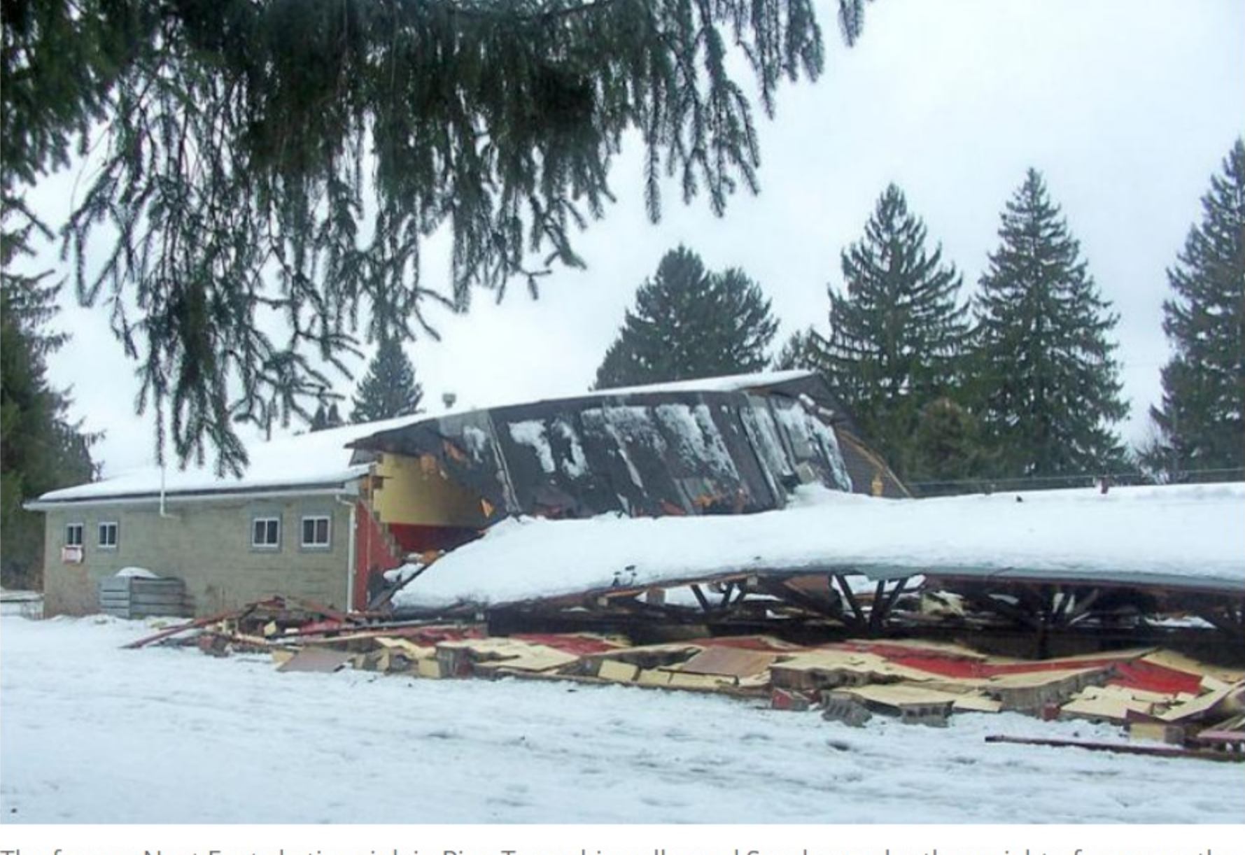
The former Neat Feat skating rink in Pine Township collapsed Sunday under the weight of snow on the roof of the vacant building.
