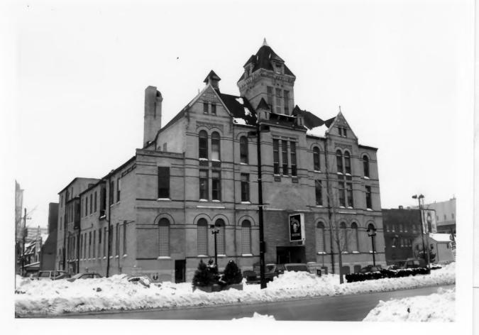
The Milwaukee Turners faces West. Note the glass block windows which cover stained glass windows seen only from the inside. The three stories on the left were added about 10 years after the original construction and are cantilevered to the main building.
