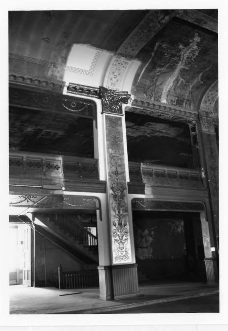
North pillar, ceiling and cornice restored by Michael DeFeber in 1987. The painting on the pillar is done on a piece of fiber glass and is identical in design to the original. The cornices are wooden with the design in plaster.
